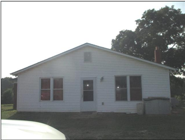
Rear view of the house
