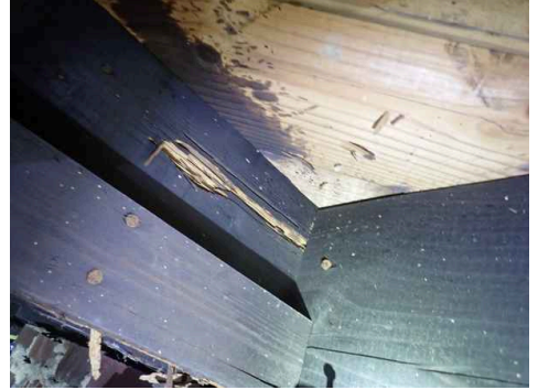
At middle chimney
