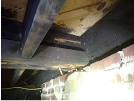
At middle chimney
