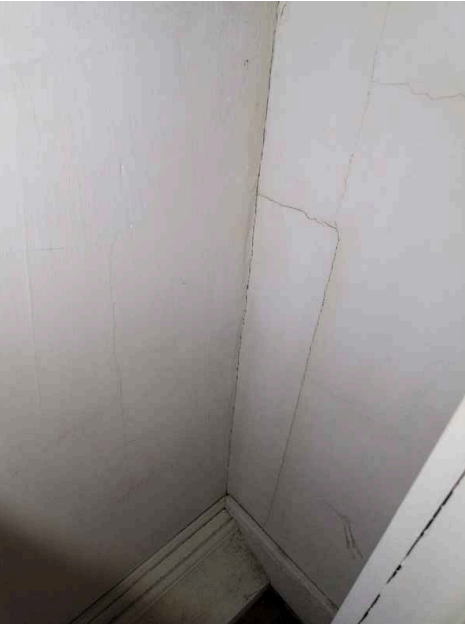
2nd Floor Right Bedroom Closet
