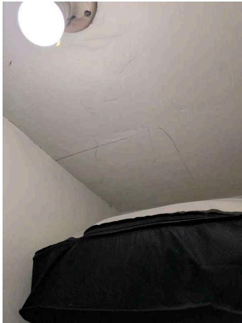
1st Floor Front Bedroom Closet
