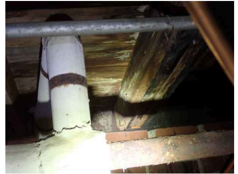
Under 1st Floor Bathroom
