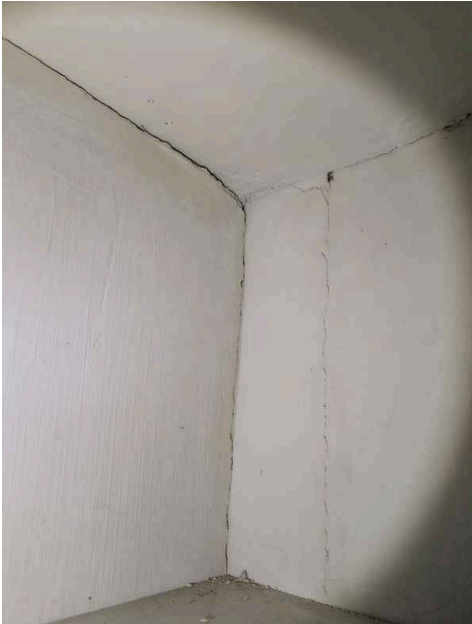
2nd Floor Right Bedroom Closet
