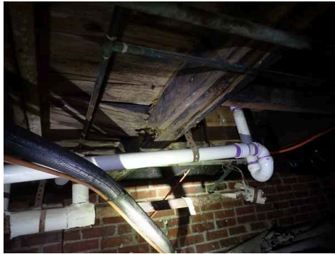
Under 1st Floor Bathroom
