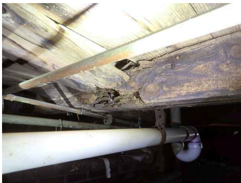
Under 1st Floor Bathroom
