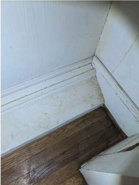
2nd Floor Right Bedroom Closet
