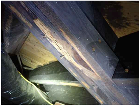
At middle chimney
