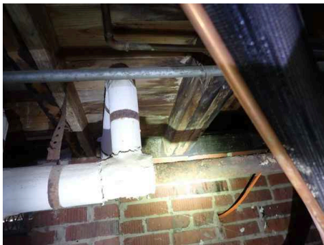
Under 1st Floor Bathroom
