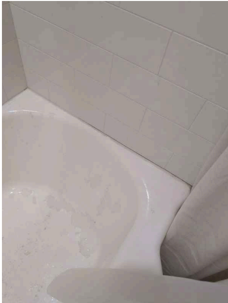
1st Floor Bathroom
