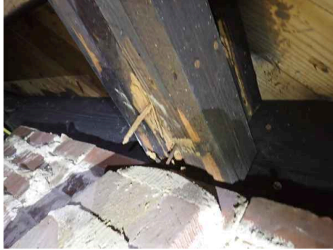
At middle chimney
