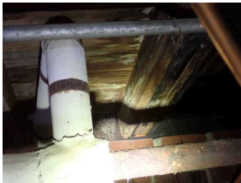
Under 1st Floor Bathroom
