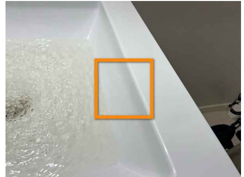
Noted at Main Bedroom
