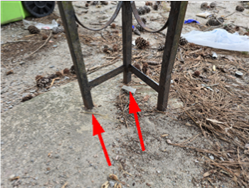
Additional Photograph: This is a photograph of above noted item 1-3
