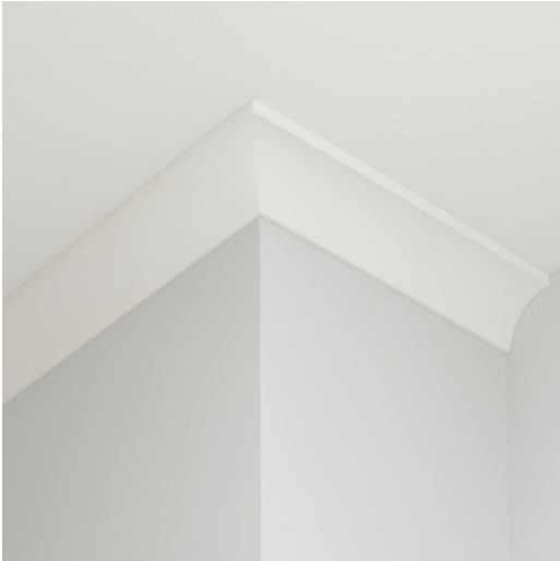
1st Floor Crown Molding Example
