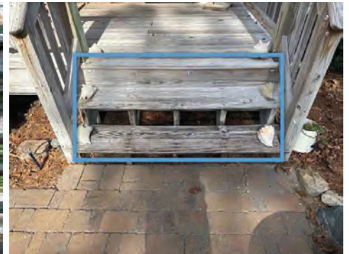
1st Floor Front Porch
