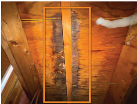
Front Right Eaves Storage
