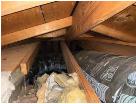
Front Left Attic
