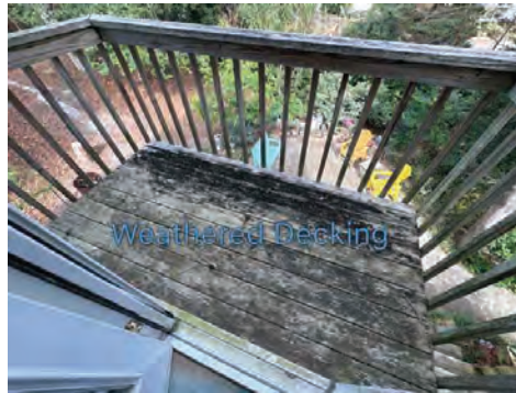
2nd Floor Rear Balcony
