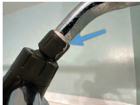
2nd Floor Rear Left Bathroom
