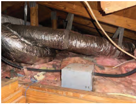
Rear Left Attic
