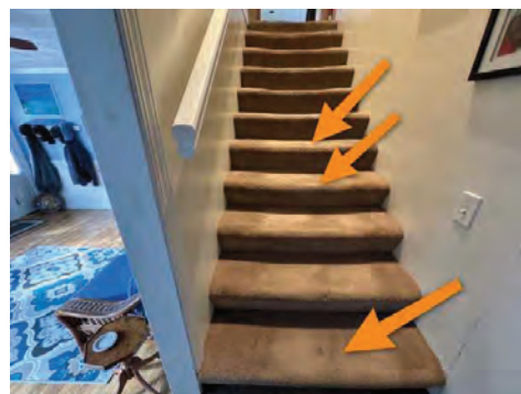
Stairs 1st to 2nd Floor
