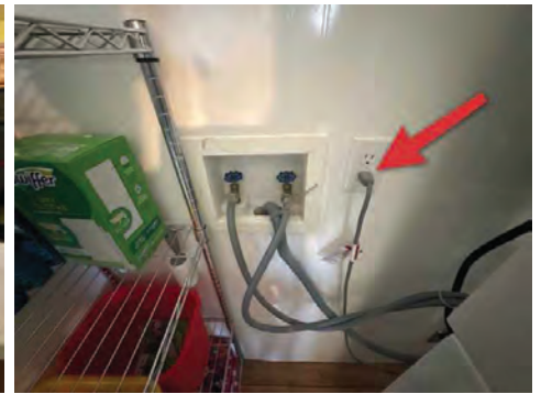
2nd Floor Laundry Room
