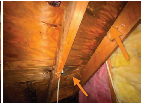
Front Right Eaves
