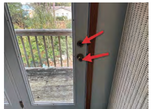
2nd Floor Rear Balcony
