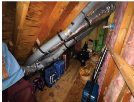
Front Right Eaves Storage
