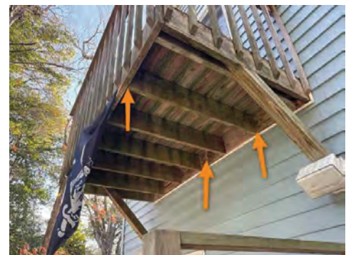
2nd Floor Rear Balcony
