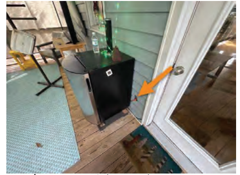
1st Floor Rear Right Porch
