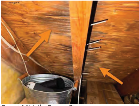
Front Middle Eaves Storage
