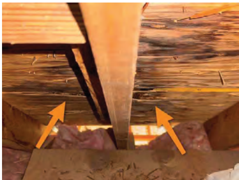
Front Right Eaves Storage
