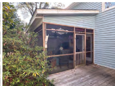
1st Floor Rear Right Porch
