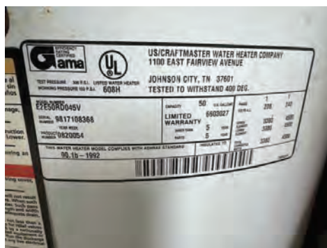
Water Heater Data Plate
