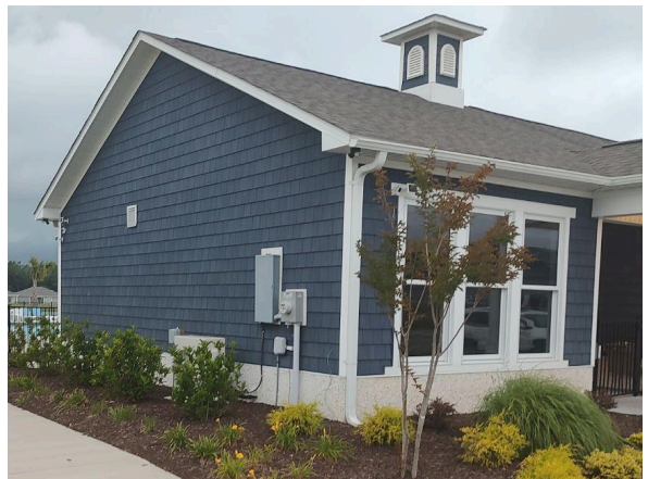
Pool house roof and exterior siding
