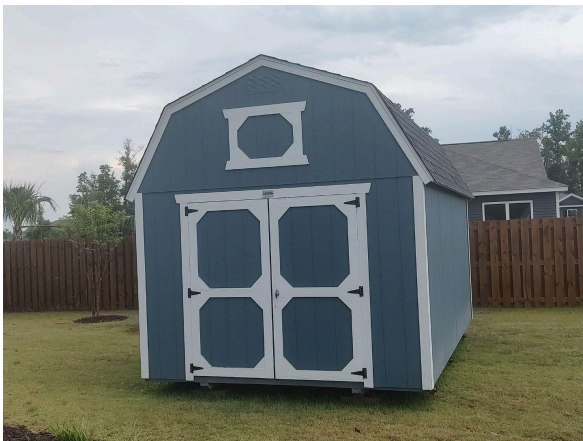
Storage building at the pool area
