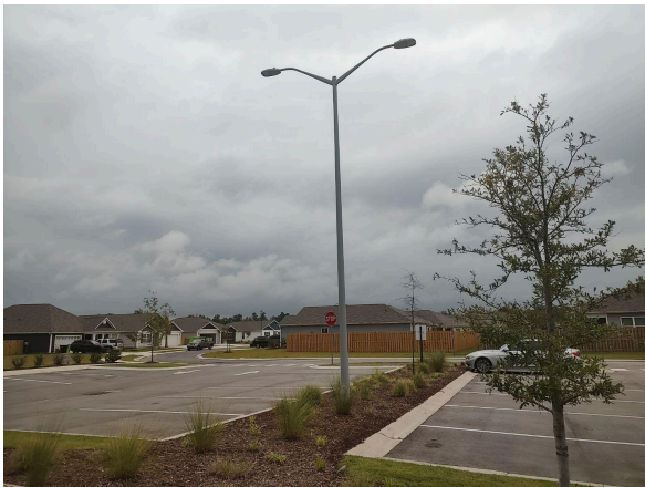
Asphalt parking area
