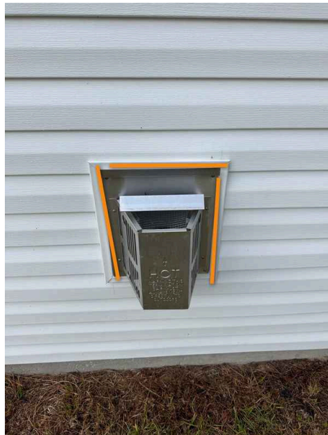
Rear - vent to J channel transition
