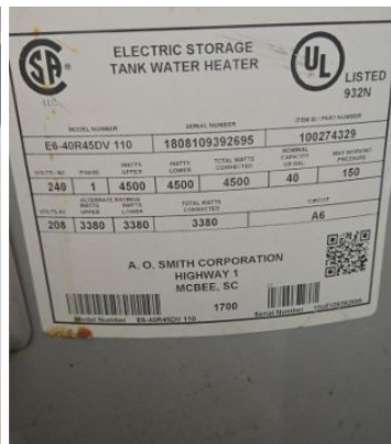
The serial number format suggests this unit was likely manufactured in August 2018
