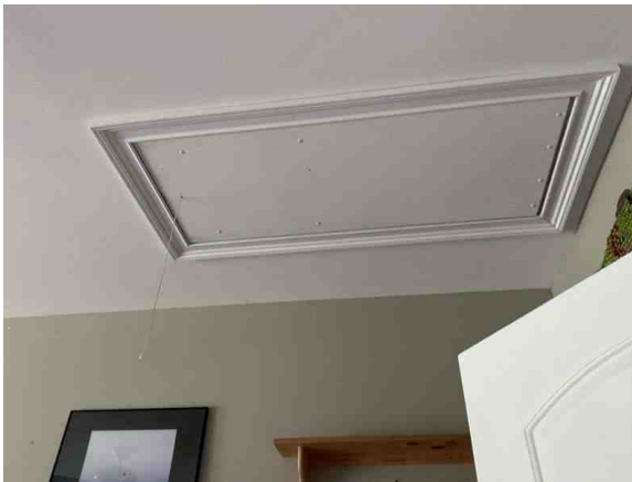
Scuttle to Attic
