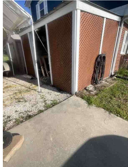
Provide sufficient clearance between the ground and any non-treated material on the covered patio enclosure
