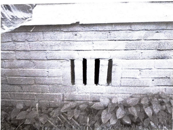
TYPICAL FLOOD VENT
