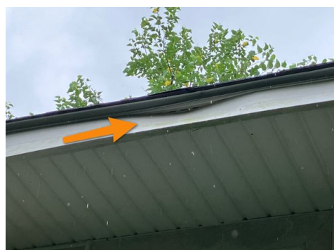
Aluminum cladding on fascia left side
