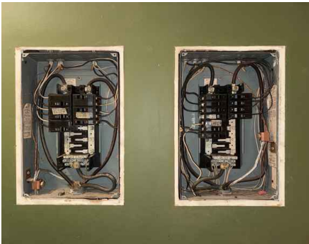
Electrical panels inspected
