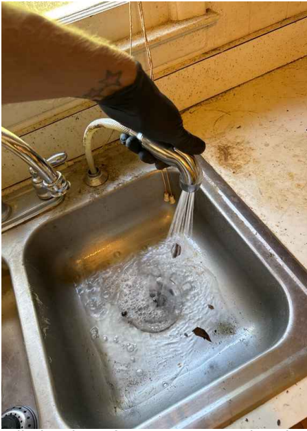
All plumbing fixtures operated and inspected
