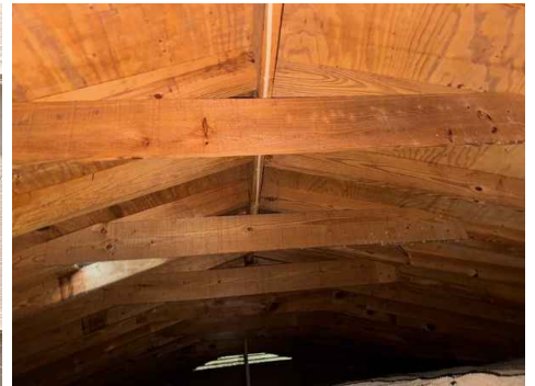
Roof deck inspected from attic
