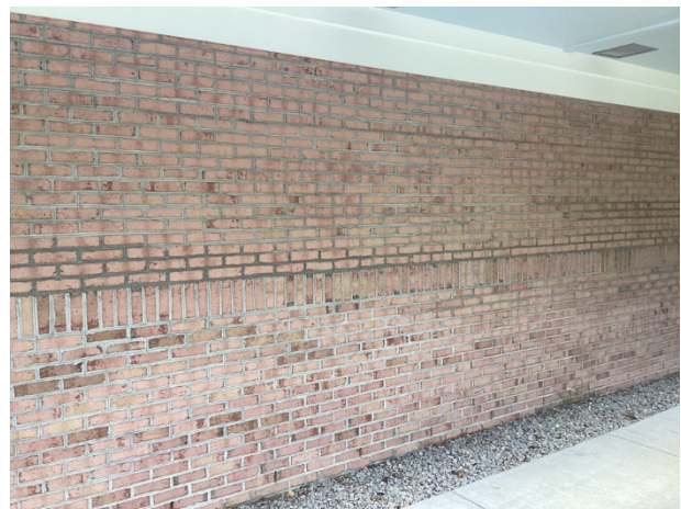
Masonry walls overview
