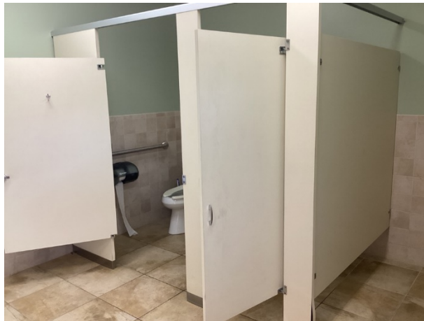
Rest room overview
