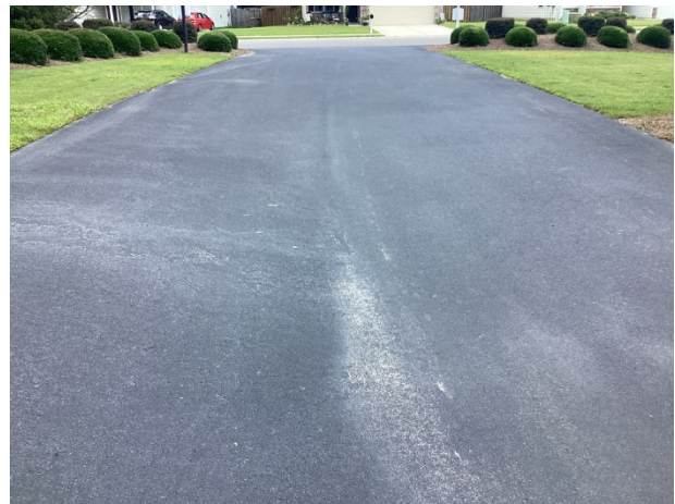
Asphalt pavement parking lot overview
