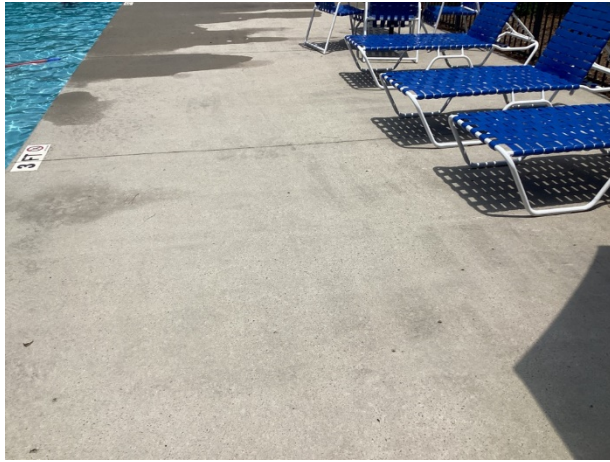
Concrete pool deck overview
