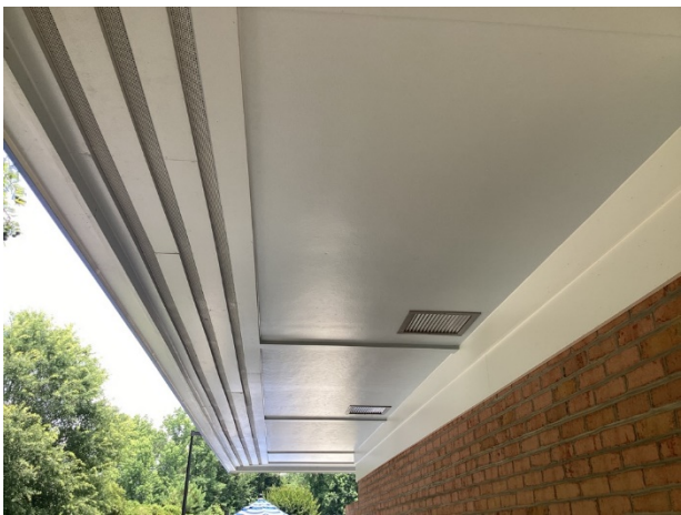
Wood soffit and fascia
