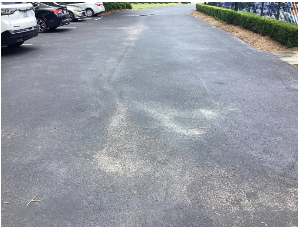
Asphalt pavement parking lot overview
