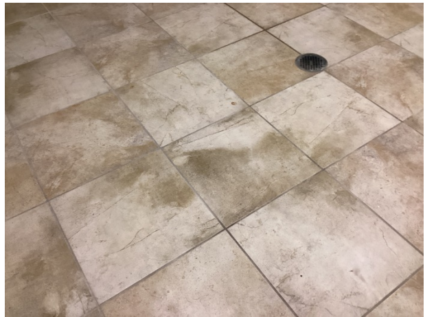
Tile floor at pool house rest room
