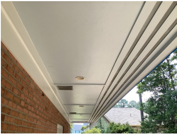
Wood soffit and fascia
