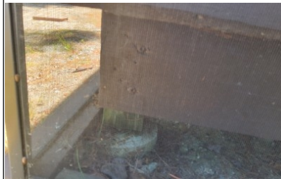
Porch is supported by concrete footings
