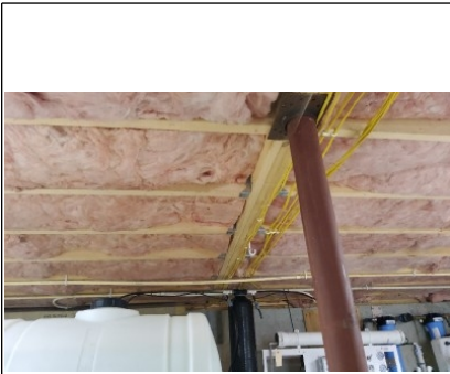
Girder and supports
