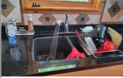
Sink and faucet
