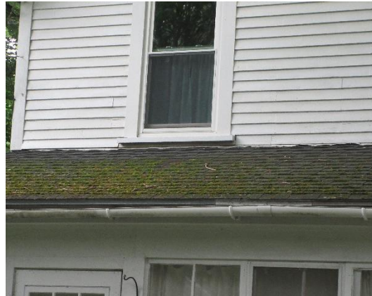
remove moss from roof
