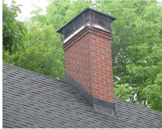
top of chimney
