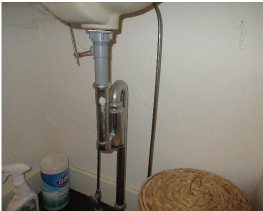
first floor 1/2 bath; plumbing under sink
