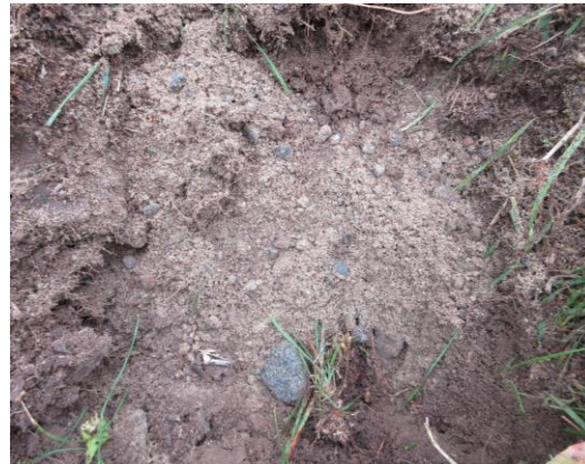
leach field excavation
