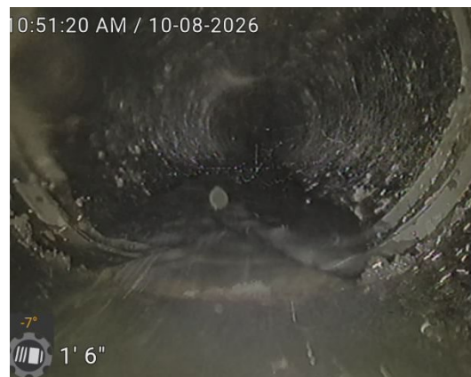
pipe to leach field
