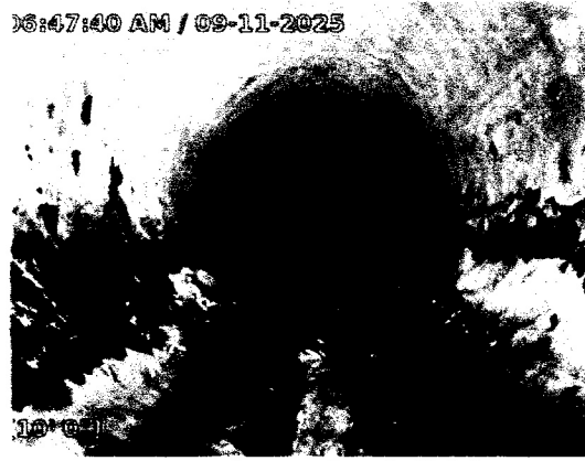
pipe to leach field
