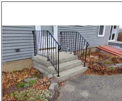
South entrance steps
