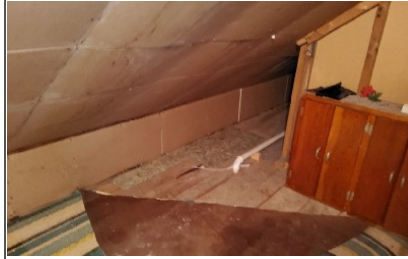
South attic eave
