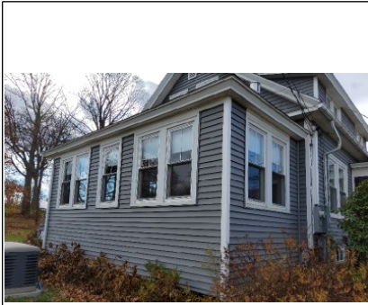
Enclosed Sun Room
