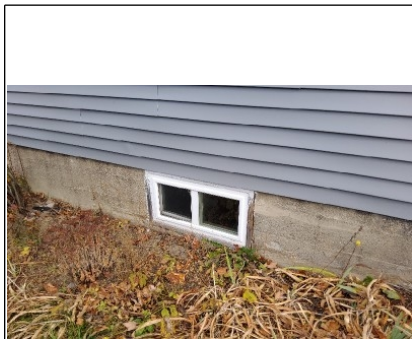
Caulk around basement windows
