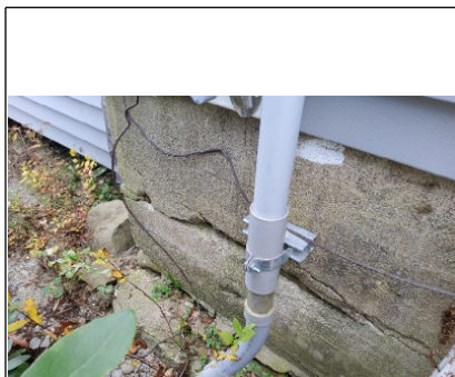
Fill cracks in along concrete stem walls to prevent further damage
