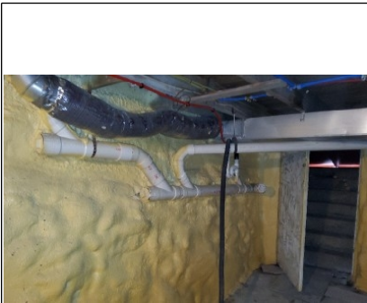
Sewer line exiting the south side of the basement
