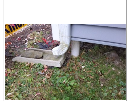
Porch supported by frost free posts
