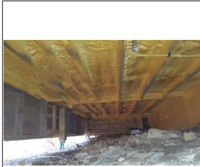
Framing has been covered with foam insulation
