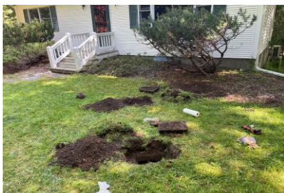
1,000-gallon concrete septic tank location
