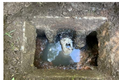
90° outlet baffle extends to tank bottom
